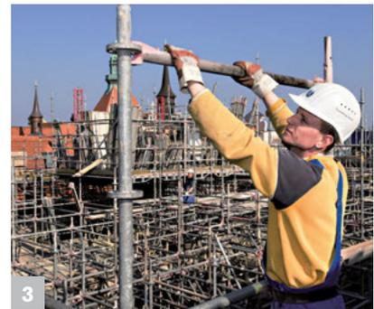
3 Safe one-man assembly in any height due to the upturned edge on the connection cups
